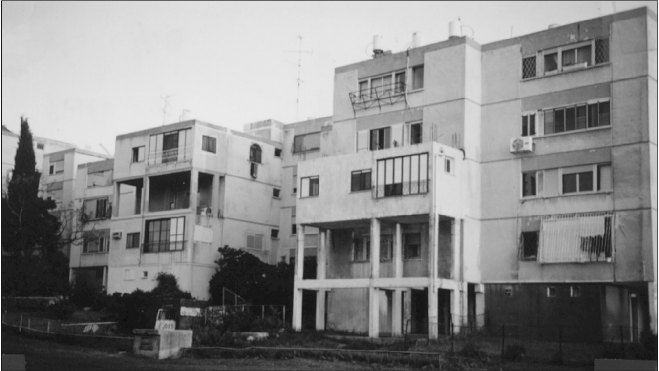
FIGURE 2. Backyard enlargements to an apartment building in Sha'ar Ha'Alyia, a moderate-income neighborhood in Haifa.
