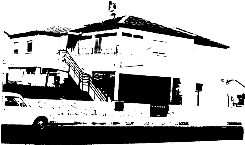
Figure 5: A Similar Four-Housing-Unit Building with Substantial Additions, Including a Private Entrance to a Second Floor Unit
