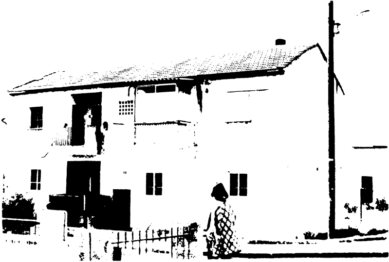
Figure 3: A Close-to-Original Building with Four Housing Units
