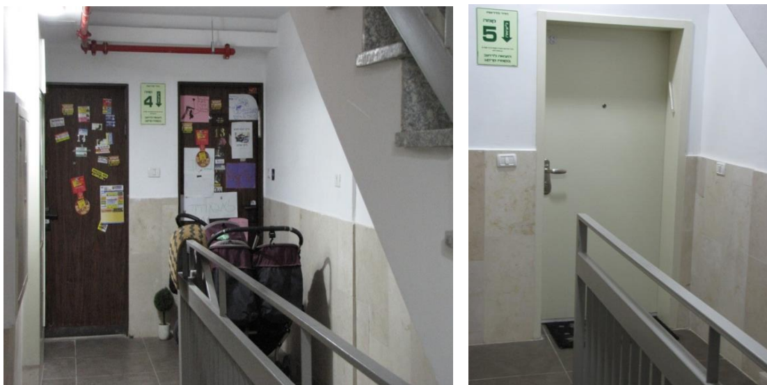
Illustration 7: Walk-up staircase in a lower floor on the left and an upper new floor on the right.
