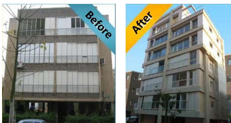
Illustration 1: One of the research buildings in Ramat Gan, before and after the renovation (Photos from the developer's website)
